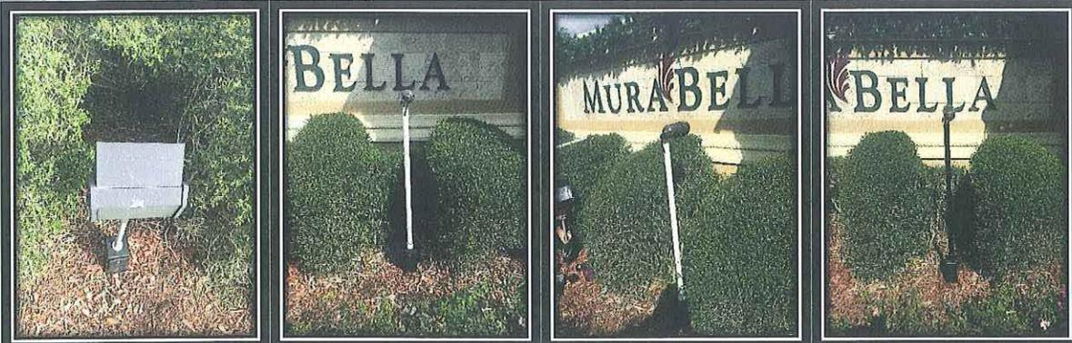
The old spot lights were rusting out and allowed moisture to get in. The bulbs kept blowing out, we replaced them with a led fixture from Home Depot.
