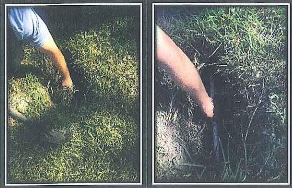
We had several broken heads, pipe and nozzles that we repaired.
